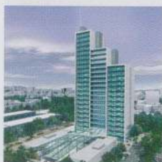
↓ | Green Tower | Desio (Mi) work in progress
