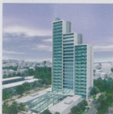
↓ | Green Tower | Desio (Mi) work in progress
